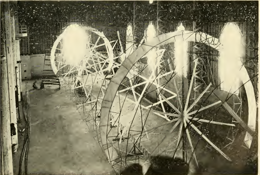
The Preble Airship Frame
