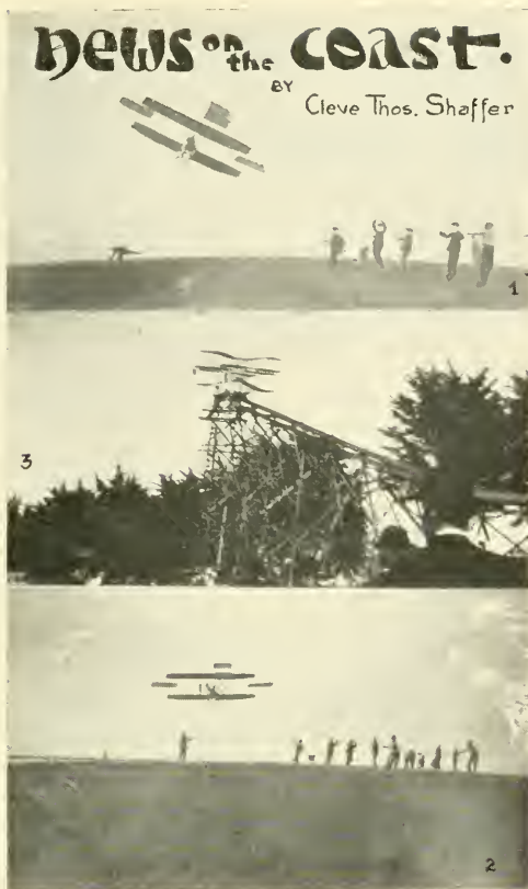
1. The Shaffer glider an instant before an accident due to breaking of both wing tips and front rudder control lever. 2. Shows machine at start of flight in which high elevation was reached. 3. Wolf-Becher gliding chute.
