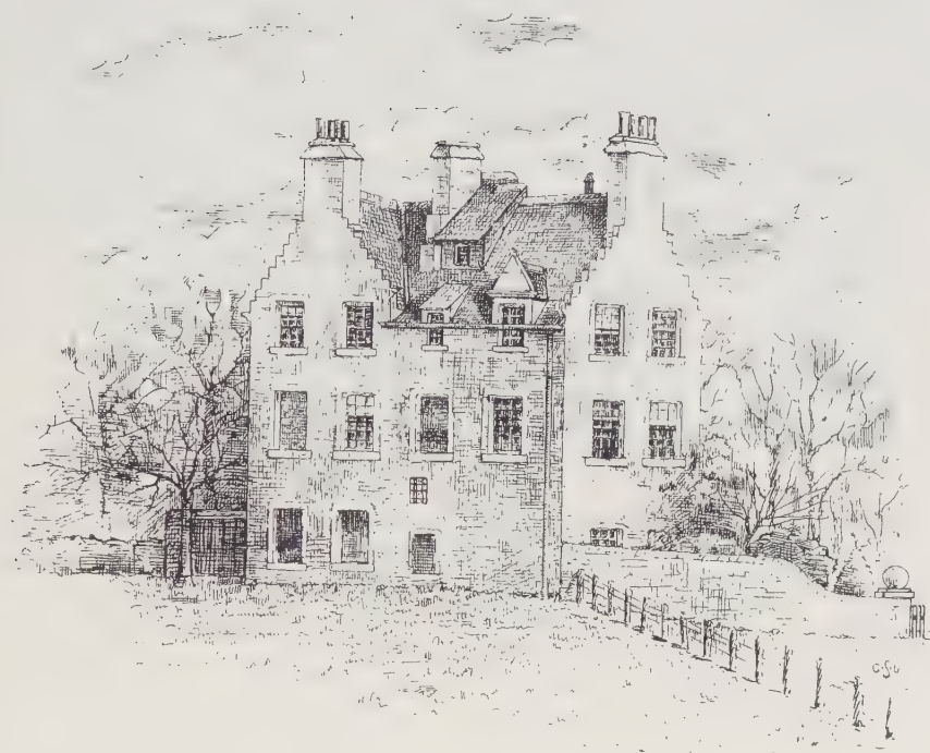
Saughton House. From the South-West.
