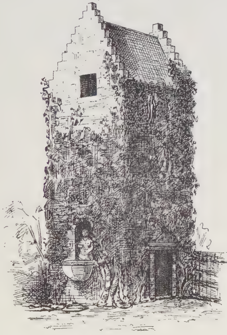
Entrance Tower Old Ravelston Ho.
