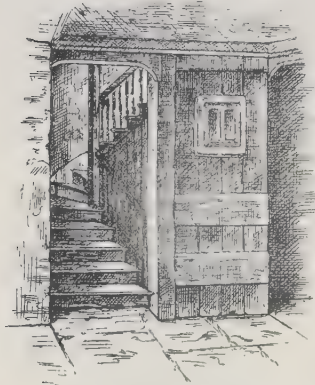
OLD STAIR, AMULREE HOUSE.
